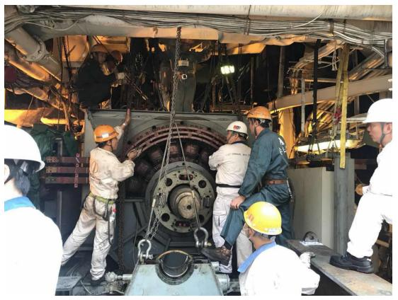
Generator's stator coil spark through; 6 insulations of generator's rotor pole coil spark through;
